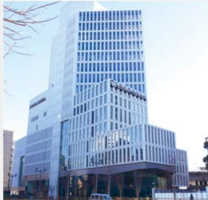
A view of Bldg. 6 from Kojimachi-Odori
