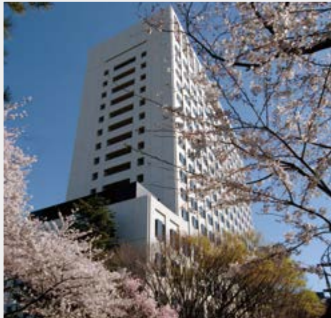
A view of Bldg. 2 from Sanadabori field
